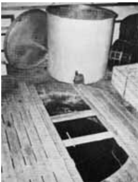
The reactor pit and alloy vessel in the Berlin-Dahlem bunker laboratory — the Virus House
