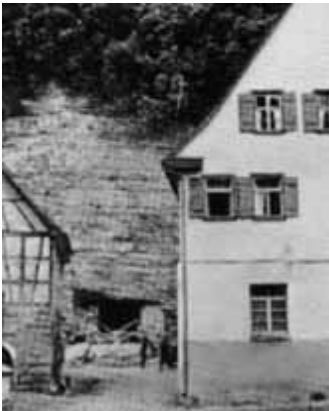
The last German atomic pile was built in a cave at Haigerloch, in southern Germany
